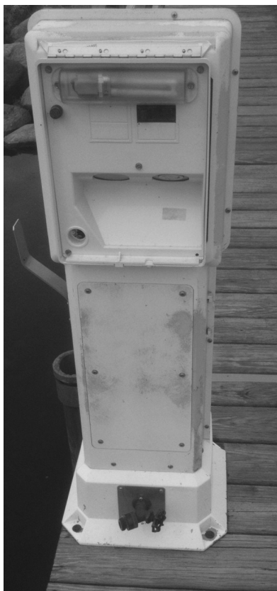
Old dock pedestal
